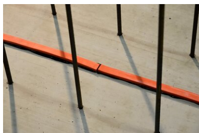
Straight butt joint
