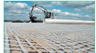
Figure 13 Secugrid® installation
