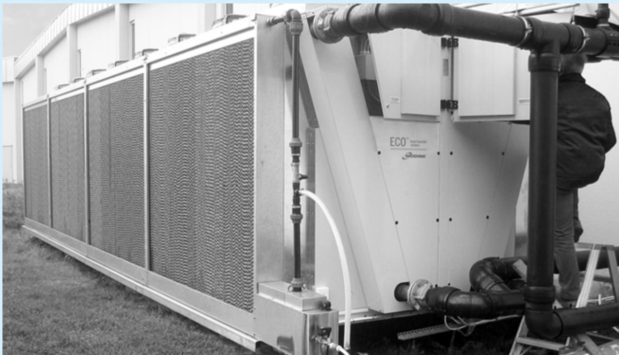
The Evaporative Panel (EEL) is installed externally on the remote condenser, gas cooler or dry-cooler. Air passes through a cellulose panel in which water partially evaporates, the water vapor is added to the air, which is at the same time cooled.
